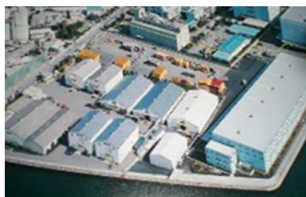
Current Overview of Tsurumi Warehouse
