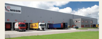
NISSIN LOGISTICS POLAND SP. Z O.O.
